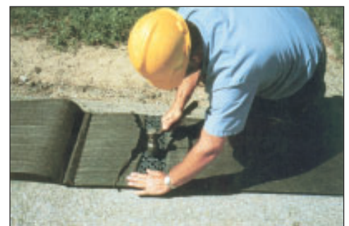
Splicing can be done by overlapping the cores and securing with a rubber hammer, overlapping the fabric and securing with underground tape.
