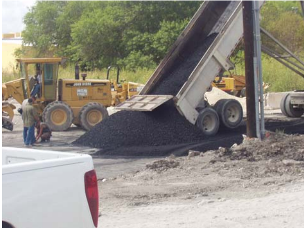
Asphalt-treated base delivery
