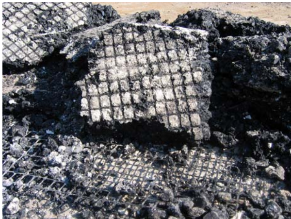
Exhumation of geogrid sample
