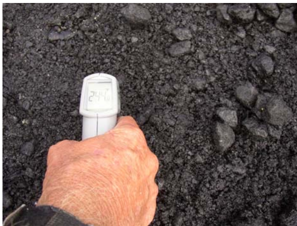
Surface reading of asphalt-treated base
