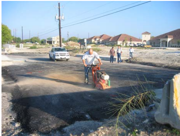
Sawcutting of black base
