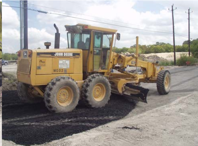
Asphalt-treated base installation
