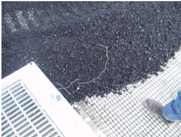
Thermocouple placement
