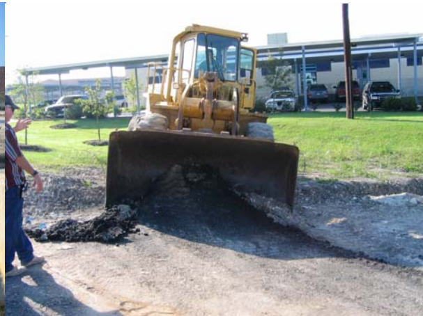
Exhumation of geogrid sample
