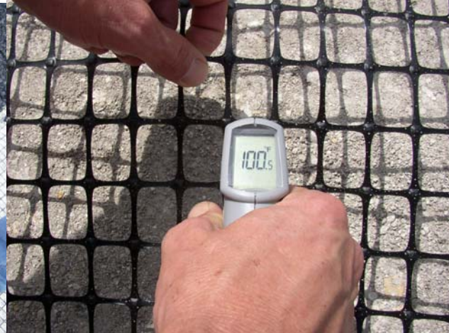
Temperature reading of subgrade
