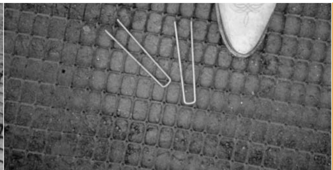
Figure 7b: Staples for anchoring BX Geogrid.
