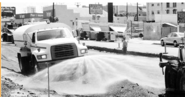
Figure 10: Moistening the fill before compaction.
