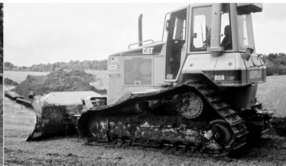
Figure 9b: Spreading aggregate fill over BX Geogrid.
