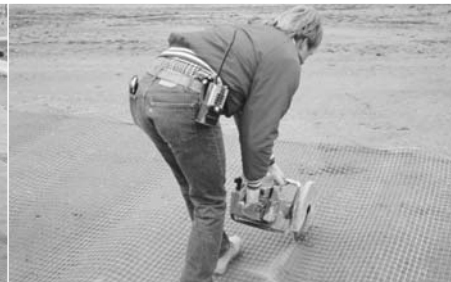
Figure 6: Using a handheld power saw to cut geogrid.
