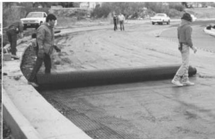
Figure 5: Placing BX Geogrid to accommodate curves.
