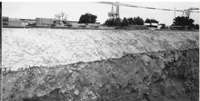
Figure 12: Geogrid can be trafficked directly by rubber-tired equipment. Figure 13: A backhoe excavation through BX Geogrid.
