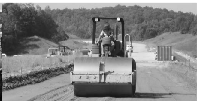
Figure 11: Compacting the aggregate fill.
