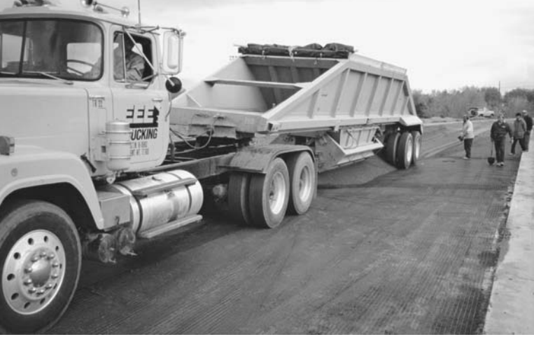
Figure 8: Dumping aggregate fill on top of BX Geogrid over competent subgrade.
