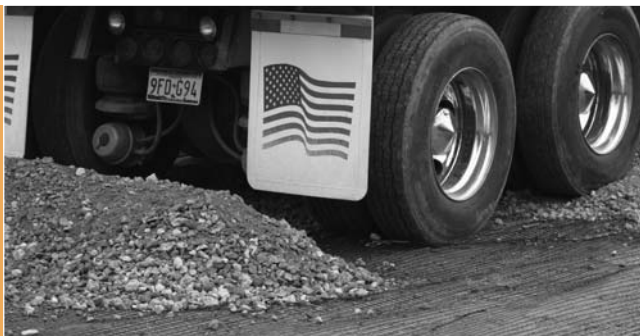
Figure 12: Geogrid can be trafficked directly by rubber-tired equipment. Figure 13: A backhoe excavation through BX Geogrid.
