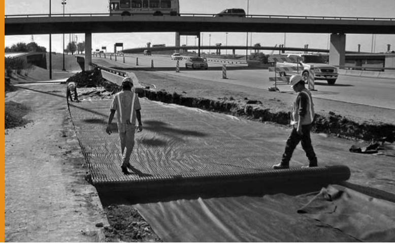
Figure 3: Rolling out Tensar BX Geogrid.
