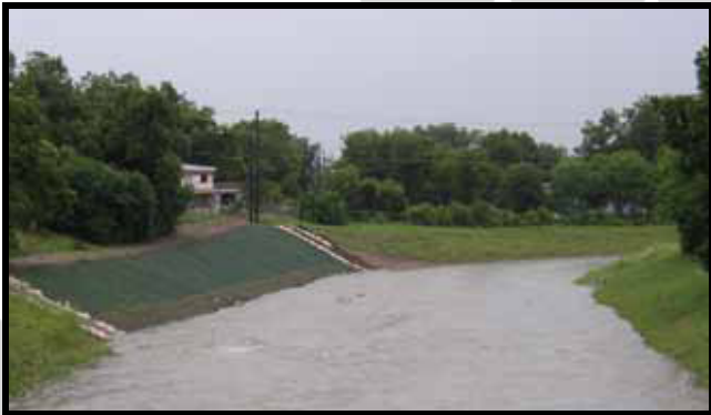
Corp of Engineers - City of San Antonio
