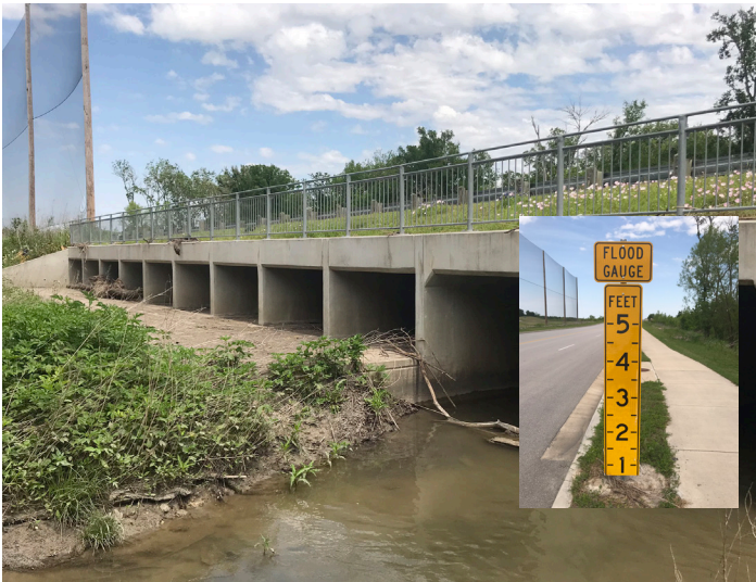
PROBLEM Scour erosion of roadway embankments during large flood events
