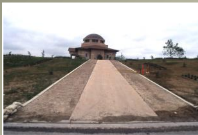
Before Lawn Seeding: GEOBLOCK paving units were installed on both sides of the paved drive for emergency access.
