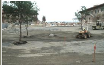
The GEOWEB cellular confinement system with engineered infill was installed in the central quad and in locations around the campus for pedestrian green walkways and emergency vehicle support.
