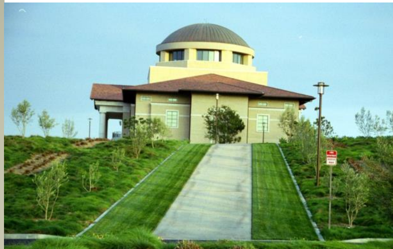
Before Lawn Seeding: GEOBLOCK paving units were installed on both sides of the paved drive for emergency access.
