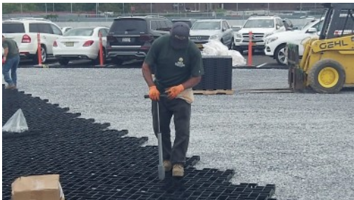
Driver utilized to install GEOPAVE U-Clip connectors for interconnected pavement.
