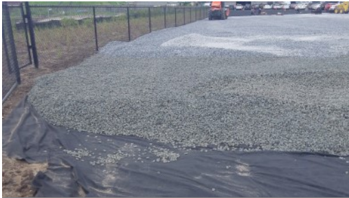
18 inches of aggregate base material was installed for stormwater retention.
