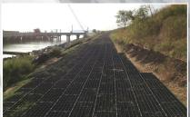
GEOTERRA Mats installed for a 15 ft. wide x 3000 ft. long roadway allow site access in an environmentally sensitive area with minimal impact.
