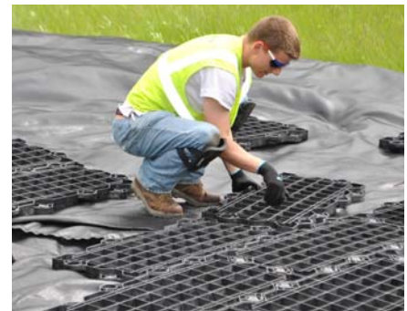
Figure 15: Placing Adjoining Units
