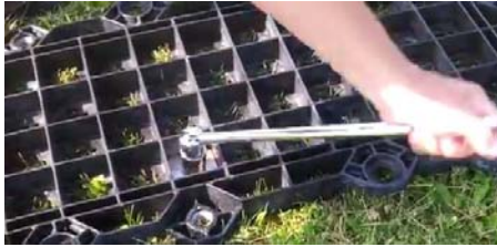
Figure 21: Auger Anchor Install with Breaker Bar
