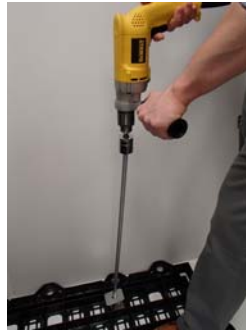
Figure 22: Auger Anchor Install with Power Drill
