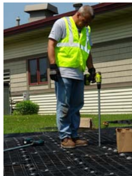
Figure 14: Installing Bolts with Power Driver
