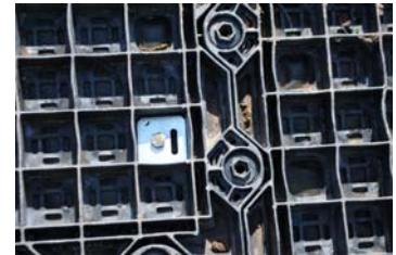
Figure 23: Installed Auger Anchor
