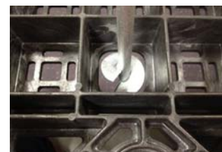
Figure 20: Insert Auger Anchor through Open Cell
