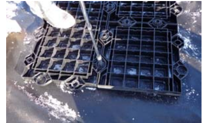
Figure 18: Final Tightening of Nuts
