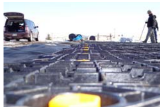
Figure 16: Yellow Bolt for Edge/Centerline Marking
