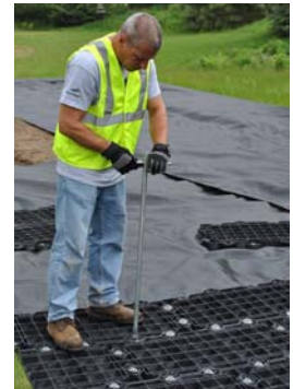
Figure 13: Installing Bolts with Manual Bolt Drive Tool
