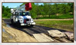
GEOTERRA Mats can be configured to fit any site requirement. GEOTERRA sections are placed over a high strength geotextile.
