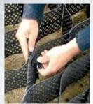
For quick and easy connection of GEOWEB® sections, exclusive ATRA® keys significantly reduce
