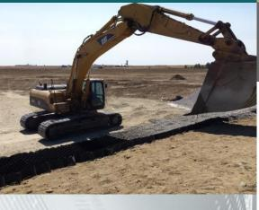
Infilling GEOWEB sections with aggregate for storm water detention pond perimeter protection.
