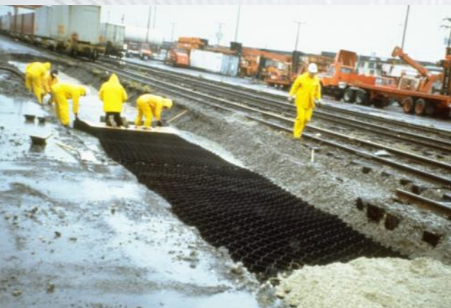
Installation of the GEOWEB sections for the FAST track testing.
