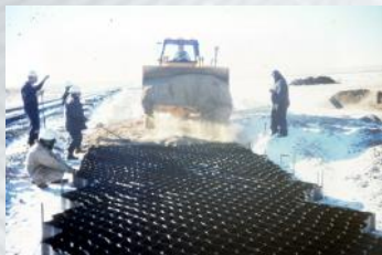
Installation of the GEOWEB sections for the FAST track testing.
