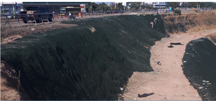
INSTALLATION LANDLOK was installed along the slopes
