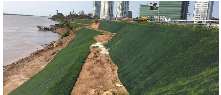
SOLUTION LANDLOK® 450 was chosen to stabilize and provide a green look to the slopes
