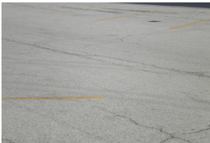
PROBLEM Excessive cracking in existing pavement
