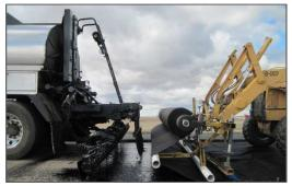
leveling course. Experienced PETROMAT installers are able to adjust the tack coat application rate within the range of 0.22 to 0.30 gallon per square yard to achieve optimum pavement performance and ease of construction. Table 1 gives the tack coat volume for one mile of road of varying widths, assuming the use of uncut paving grade asphalt tack coat.
