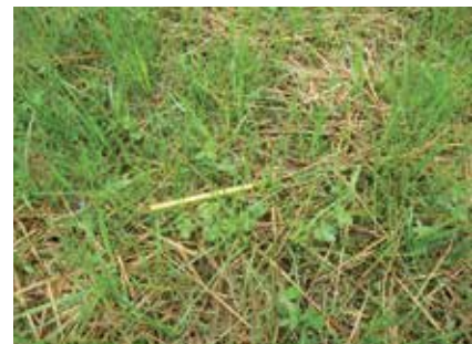
By April 17, the site had been stabilized and vegetation establishment was well underway.
