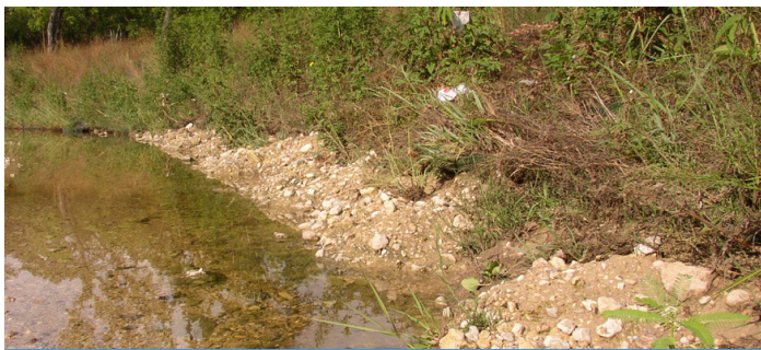
PROBLEM Severe erosion caused by an earthen channel failing during flooding
