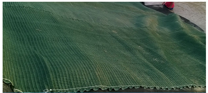
SOLUTION PYRAMAT® 75 used to stabilize and mitigate future erosion problems
