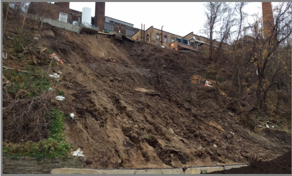
Slope prior to application, June 2014
