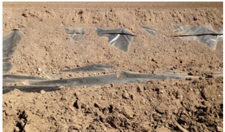
Figure 3: Soil covering the liner
