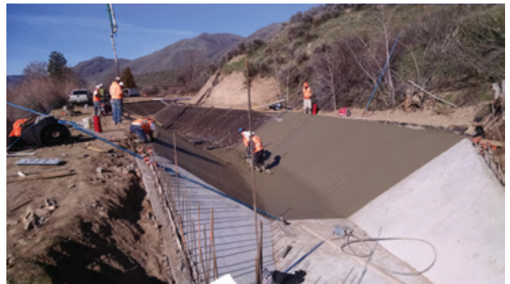
Figure 4: Reinforced concrete being poured onto ArmorPad 3NWLD
