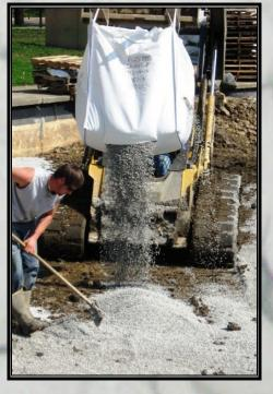
Provided the product is kept dry, AquaBlok® can be handled much like crushed stone aggregate. Conventional methods and equipment can be utilized to apply the material in a broad range of environments and circumstances.
