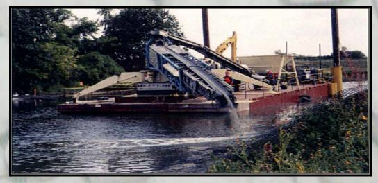
Provided the product is kept dry, AquaBlok® can be handled much like crushed stone aggregate. Conventional methods and equipment can be utilized to apply the material in a broad range of environments and circumstances.
