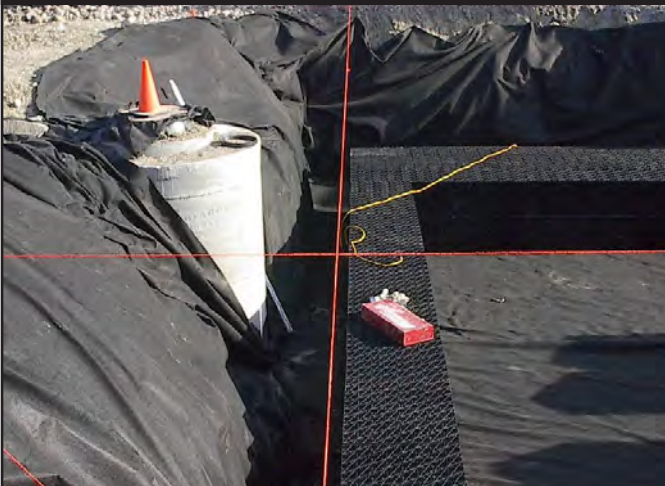
STRING LINES FACILITATE INSTALLATION OF BASE LAYER
