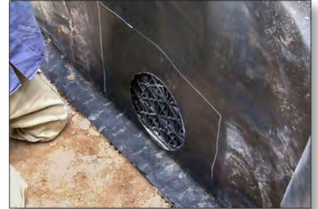
3. Cut the opening for the pipe
