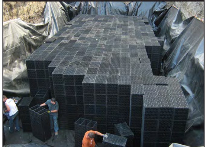
INSTALLING FLO-CELL® CAPPING LAYING OVER TANK MODULES
