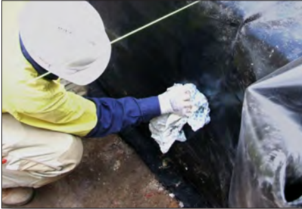
1. Clean the area where the boot is to be installed
