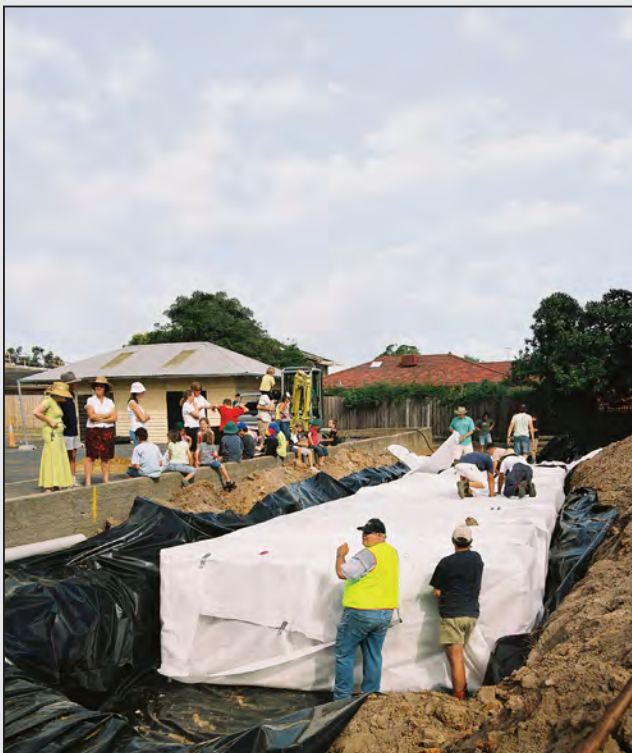
Constructed tank is wrapped in geotextile.
