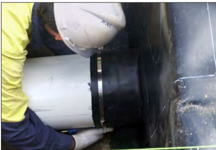
10. Move the clamp over and around the boot and tighten
