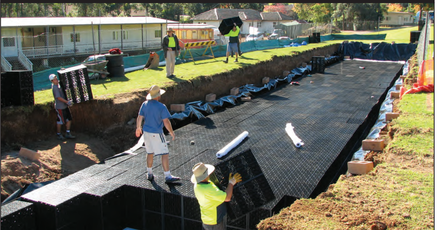
INSTALLING TANK MODULES
