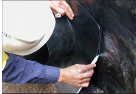
2. Trace the edge of the boot onto the tank liner
