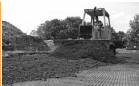
Figure 4: Geogrid should overlap in the direction of advancing fill.
