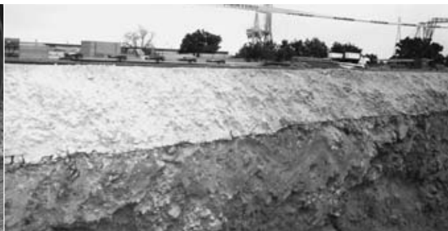
Figure 13: A backhoe excavation through BX Geogrid.
