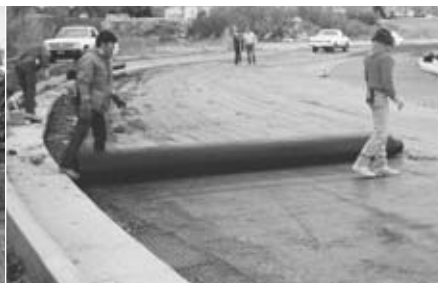
Figure 5: Placing BX Geogrid to accommodate curves.
