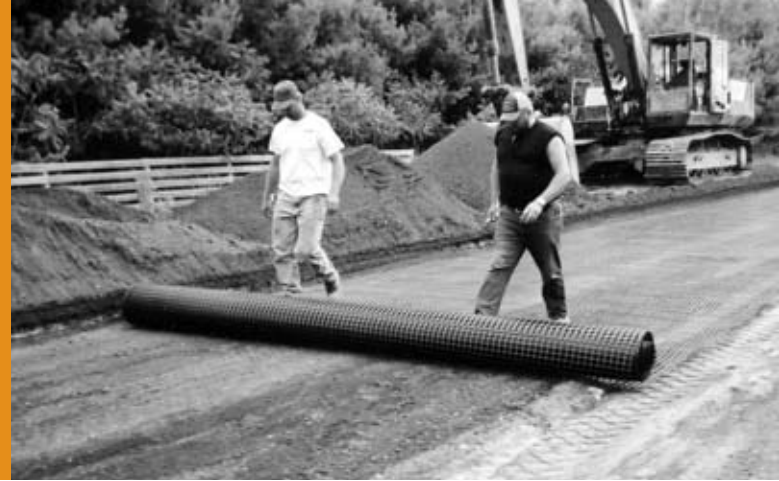
Figure 3: Rolling out the BX Geogrid.
