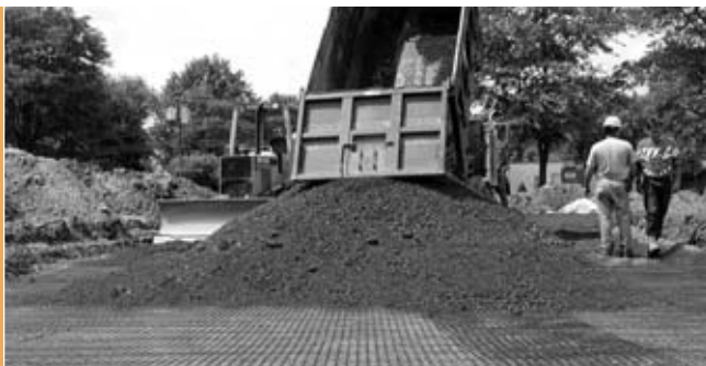
Figure 9a: Dumping aggregate fill on top of BX Geogrid over soft subgrade.
