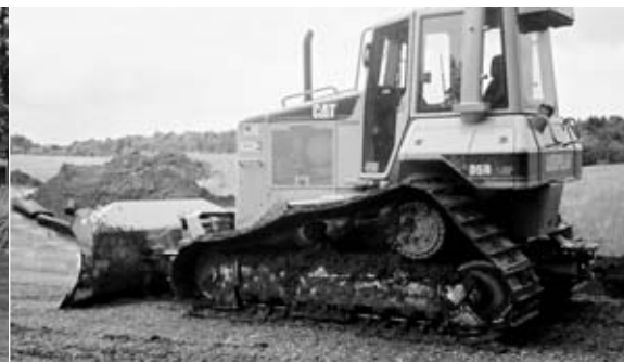
Figure 9b: Spreading aggregate fill over BX Geogrid.
