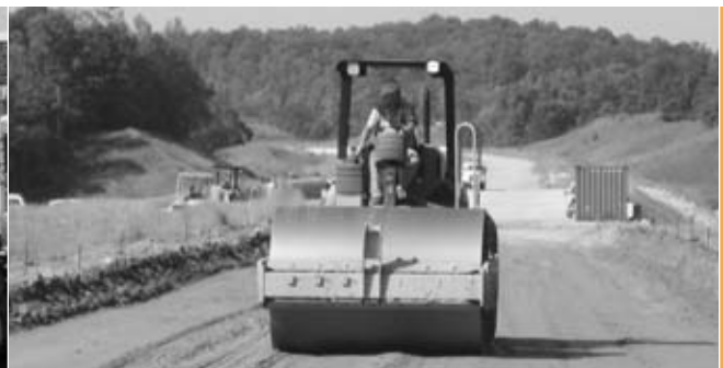
Figure 11: Compacting the aggregate fill.
