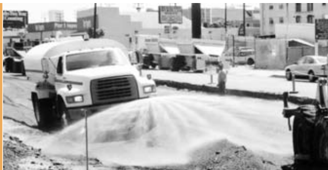
Figure 10: Moistening the fill before compaction.
