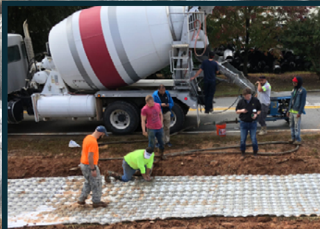
Cast-in-place installation during pumping of concrete
