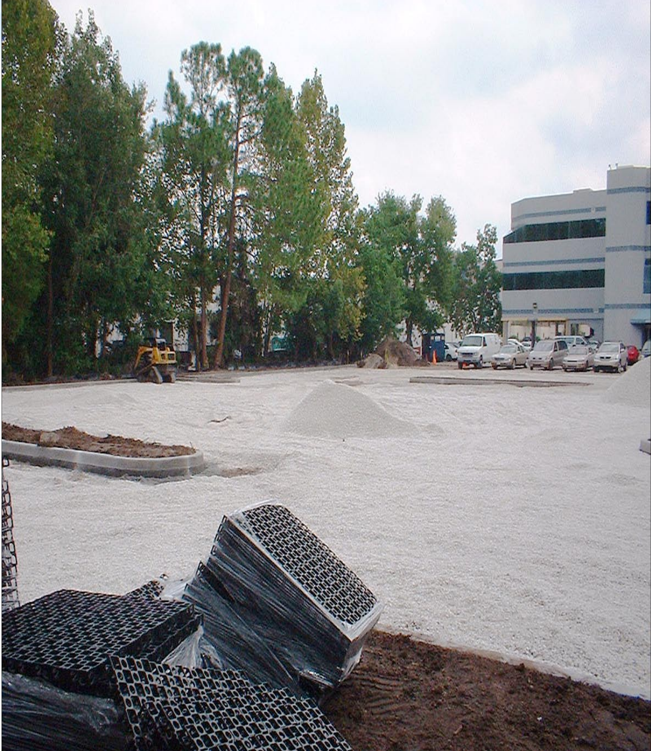
Preparing the sandy base of the Atlantis ® Turf Cell ® installation.
