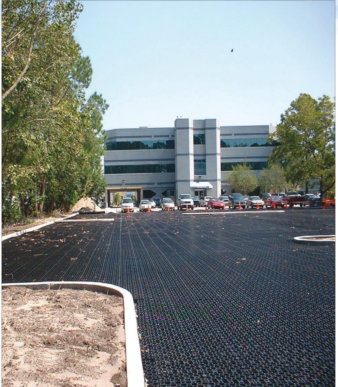
The Atlantis ® Turf Cell ® installed in place.
