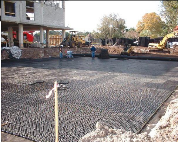
Laying of 52mm cell for underdrain.
