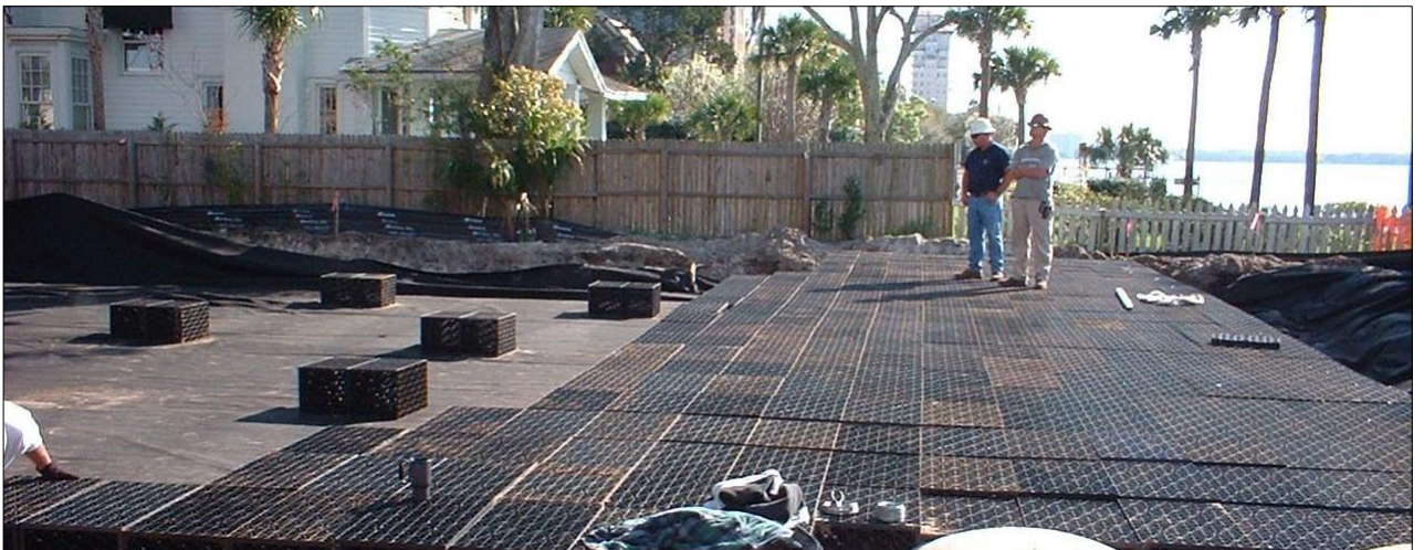
Installation of the Atlantis ® Matrix ® tank modules.
