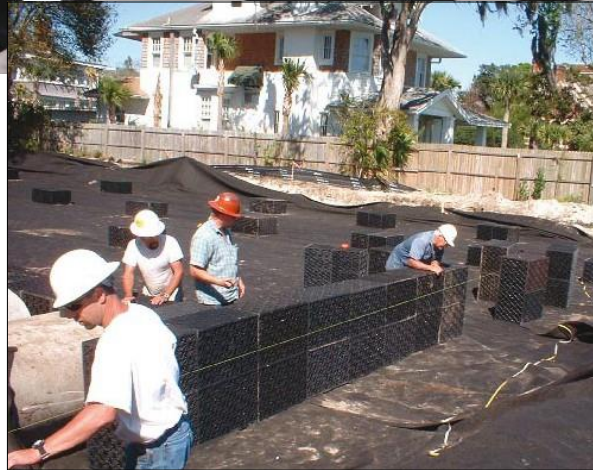
Atlantis® Matrix® double tank modules being laid into place
