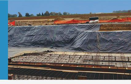
ERTHA PVC geomembranes were developed for applications such as landfills, canals, ponds and other containment purposes. They are formulated to withstand atmospheric pollutants and chemicals commonly found in industrial settings.
