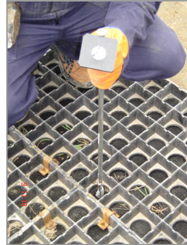
Figure 32: Installing the Earth Anchor
