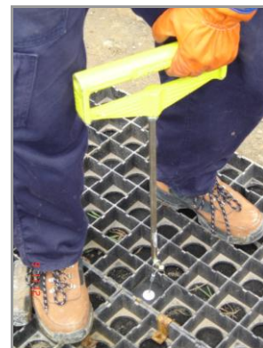
Figure 34: Setting the Earth Anchor
