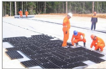
Figure 30: Placing GEOTERRA Mats Over Geotextile Layer
