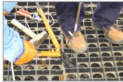
Figure 35: Crimping the Cable Stop
