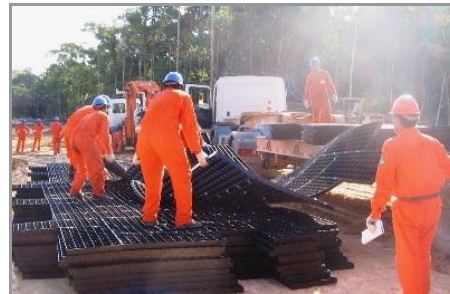
Figure 27: Transporting Pre-Assembled Mats from Off-Site
