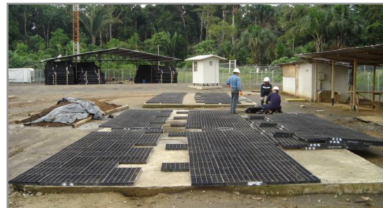
Figure 31: Connecting Pre-Assembled GEOTERRA Mats
