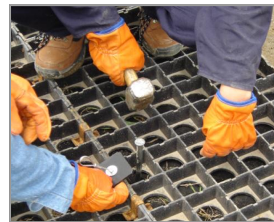
Figure 33: Driving the Anchor Head
