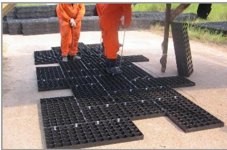
Figure 28: Assembling GEOTERRA Mats (Herringbone Pattern)
