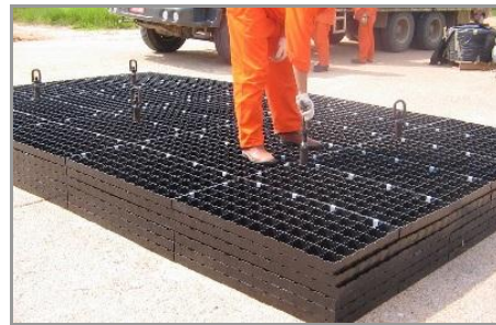
Figure 29: Assembling GEOTERRA Mats (Side-by-Side Pattern)
