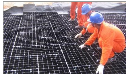
Figure 16: Connecting GEOTERRA Units
