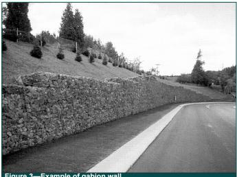
Figure 3—Example of gabion wall
