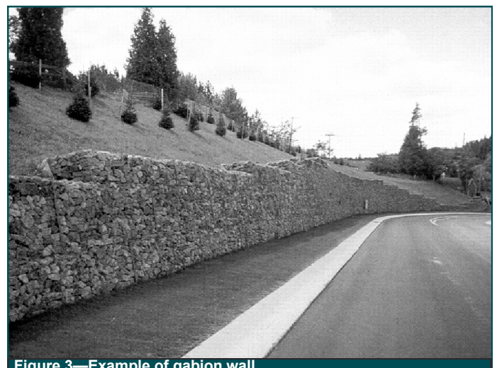
Figure 3—Example of gabion wall
