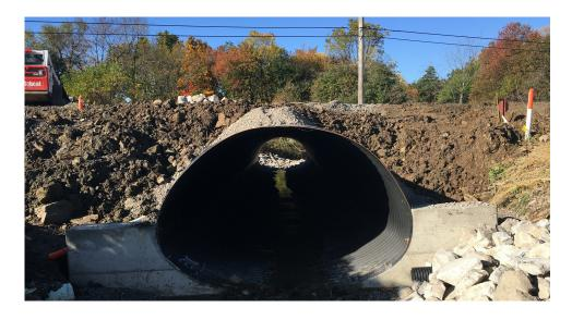
In Huron County, an older storm culvert needed replacement along State Route 601 near Norwalk, Ohio. The Ohio Department of Transportation (ODOT) reviewed options and selected a HEL-COR<sup>®</sup> CMP culvert manufactured by Contech Engineered Solutions to replace the existing, deteriorated culvert. HEL-COR<sup>®</sup> CMP was an approved product and would meet both the structural and sizing requirements.
