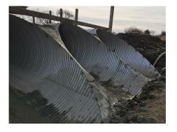
specifically designed to prevent scour, and the pipe was also rotated at a 10 degree skew to help with channel alignment.
