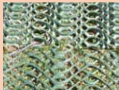
Mesh 'Butt' joined using U-pins
