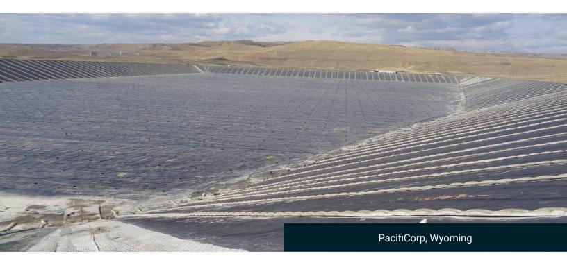
HYDROTEX® 4" CONCRETE BALLAST BLOCK (CBB400) Installation was pumped in place in 20 ft intervals
