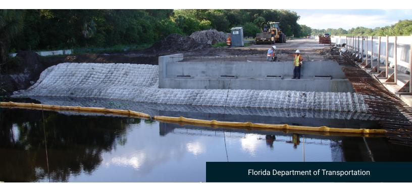
HYDROTEX® 4" ARTICULATING BLOCK (AB400) Installation was locally pumped then lifted into place
