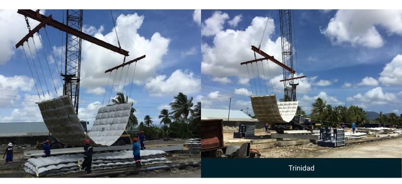
HYDROTEX® 12" ARTICULATING BLOCK (AB1200) Installation was locally pumped then lifted into place
