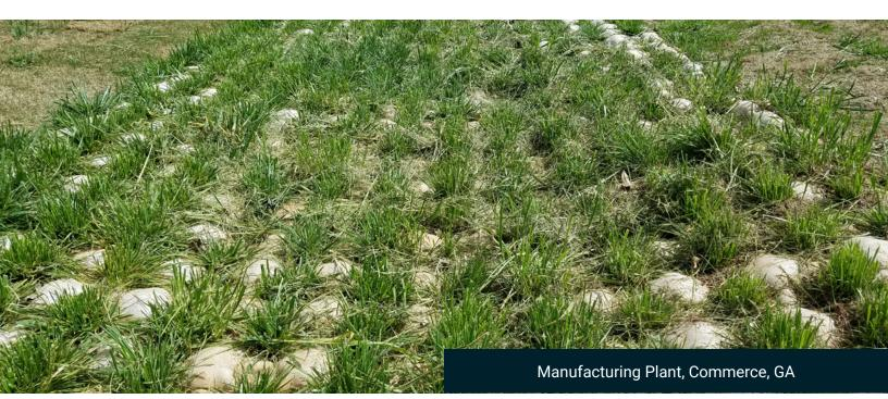
HYDROTEX® 1" ENVIROMAT FX (FX100) - U.S. AND FOREIGN PATENTS PENDING Installation was pumped in place over a double net straw mat
