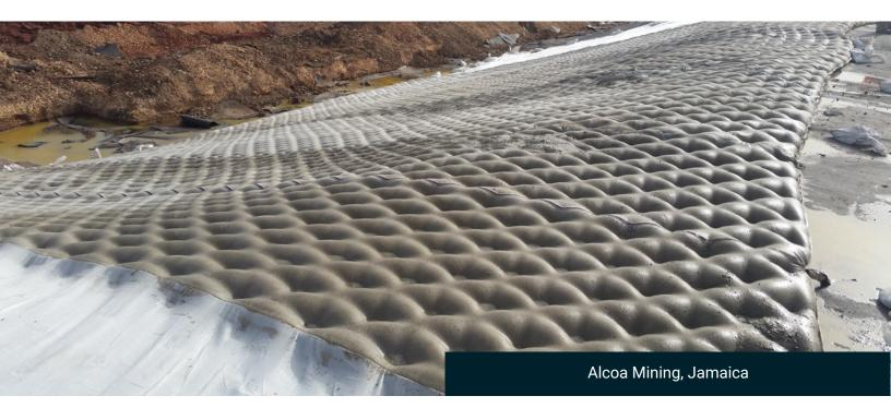
HYDROTEX® 6" FILTER POINT (FP600) Installation was pumped in place over a permanent liner
