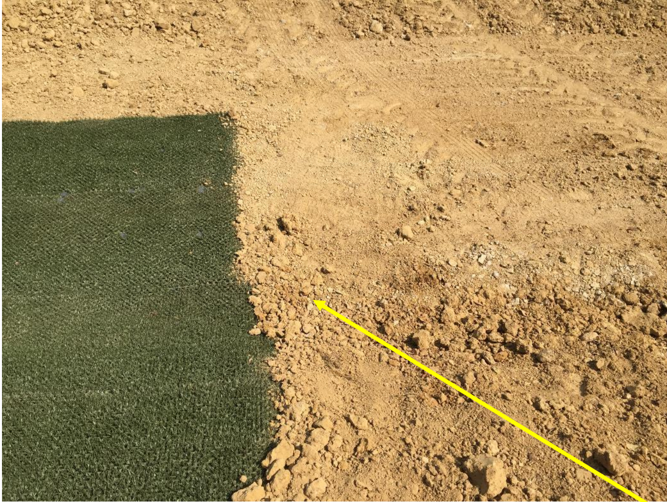
Upslope terminal ends of mats were trenched in approximately 6 inches (left). Mat edges at top of both sideslopes (Right photo) and downstream terminal ends were simply stapled on 9 inch centers with loose soil placed over edges.
