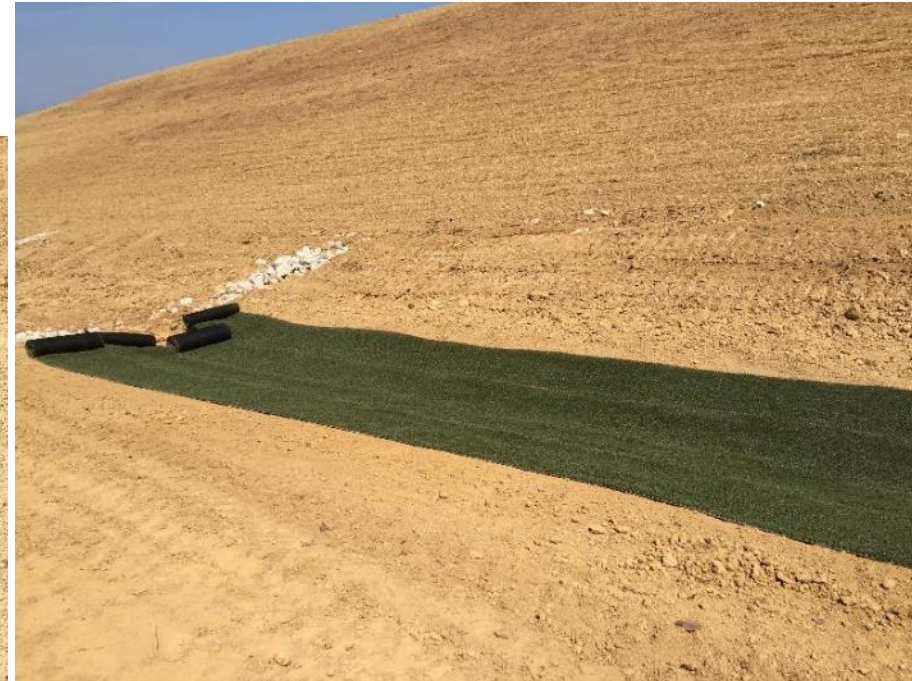
ShearForce10 Installed over cool season grass mix in high flow channel at the base of an overburden cap on September 10, 2019. Objective: Evaluate potential as rock riprap replacement in high flow areas.
