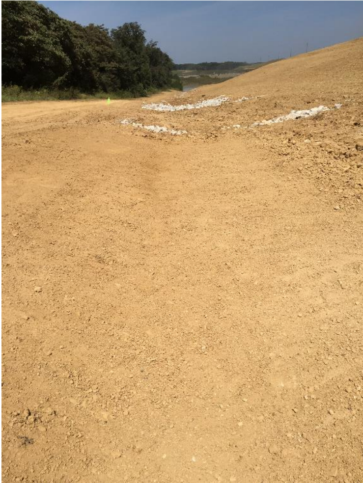
ShearForce10 Installed over cool season grass mix in high flow channel at the base of an overburden cap on September 10, 2019. Objective: Evaluate potential as rock riprap replacement in high flow areas.
