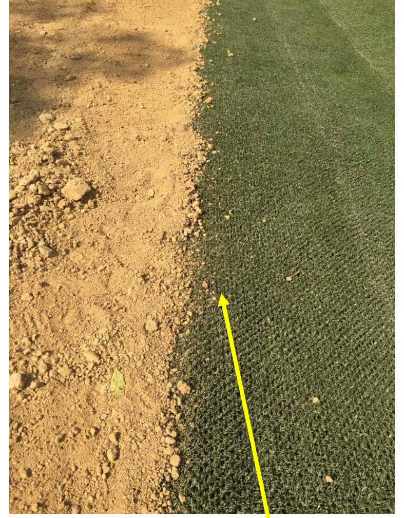
Upslope terminal ends of mats were trenched in approximately 6 inches (left). Mat edges at top of both sideslopes (Right photo) and downstream terminal ends were simply stapled on 9 inch centers with loose soil placed over edges.
