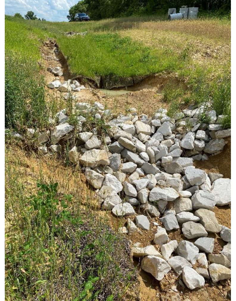
May 28, leveled rock check dam
