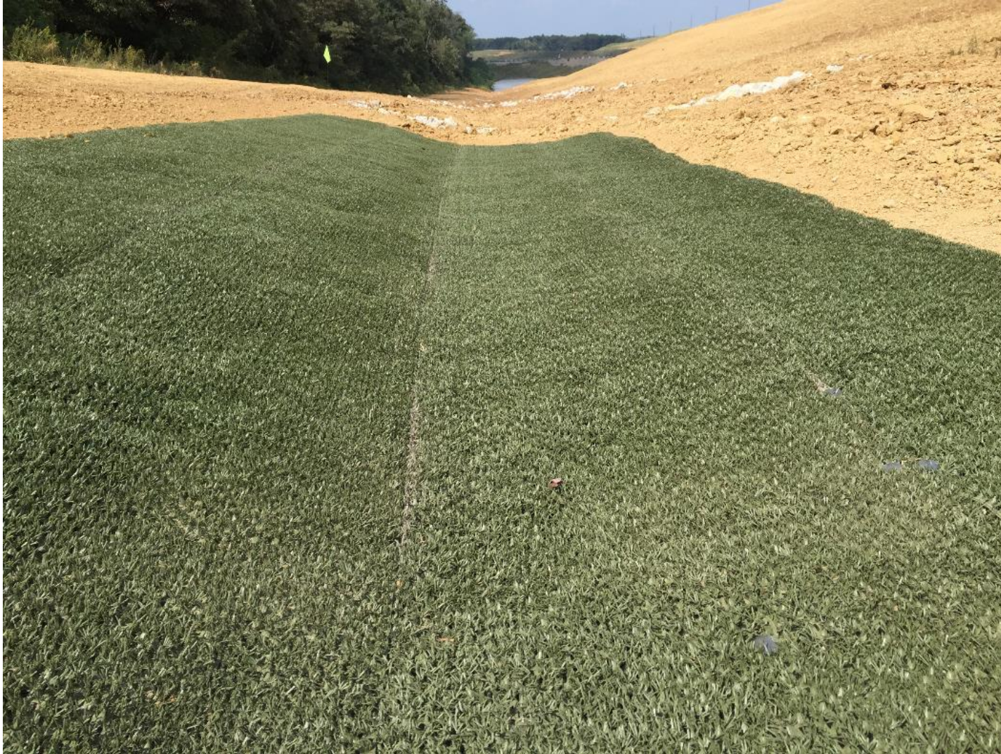
Completed ShearForce10 Installation looking down channel grade
