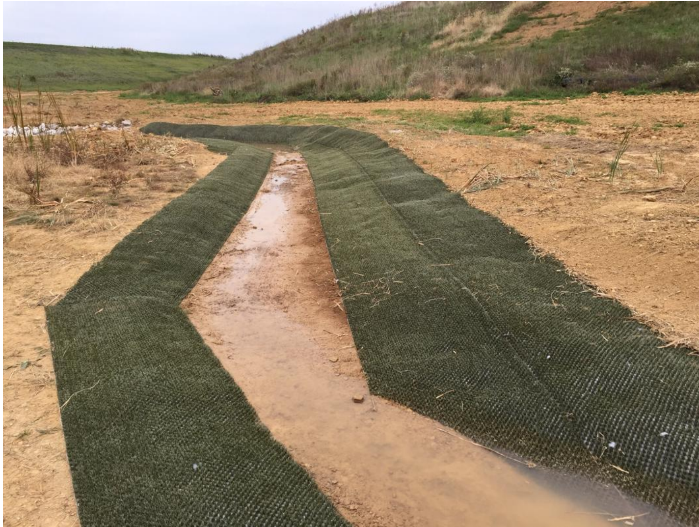
InstaTurf ShearForce10 Instant Armor Mat Installed October 25, 2018 on seeded streambank
