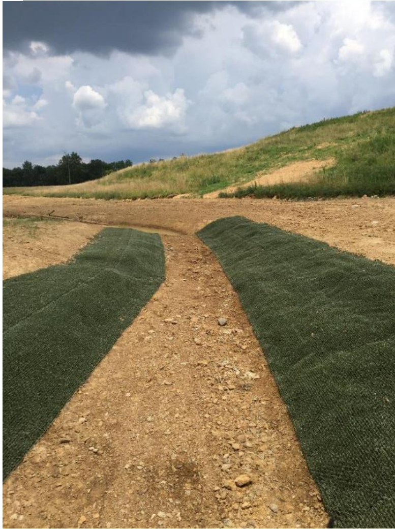
ShearForce10 just after installation on June 28, 2019 (left). 2 months after installation, vegetation developing nicely (right).
