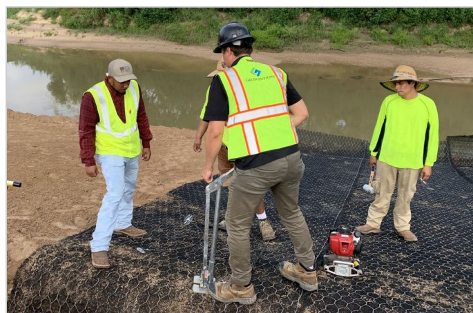
Installing the anchors
