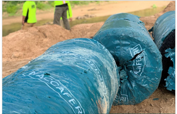
Materials on site - Ready to Begin
