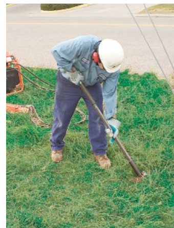
3. Pull the drive steel out of the ground.
