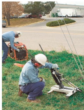
5. The portable power source operates the Load Locker which grips the adapter setting bar and rotates the anchor underground into position. The desired holding capacity is set with the Load Locker gauge.
