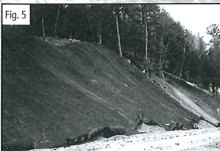
After installation and before vegetation
