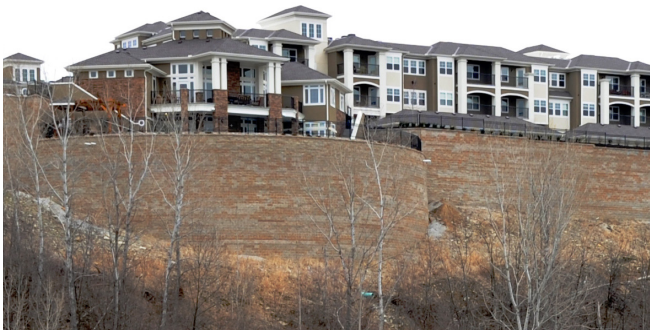
The corrosive resistant properties of Tensor Geogrids allowed the use of recycled concrete for the backfill material, providing overall project savings.
