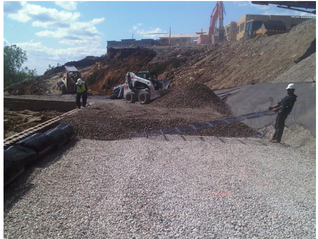
Inert to chemical degradation, Tensar HDPE Geogrids are able to withstand the high alkalinity found in recycled concrete.
