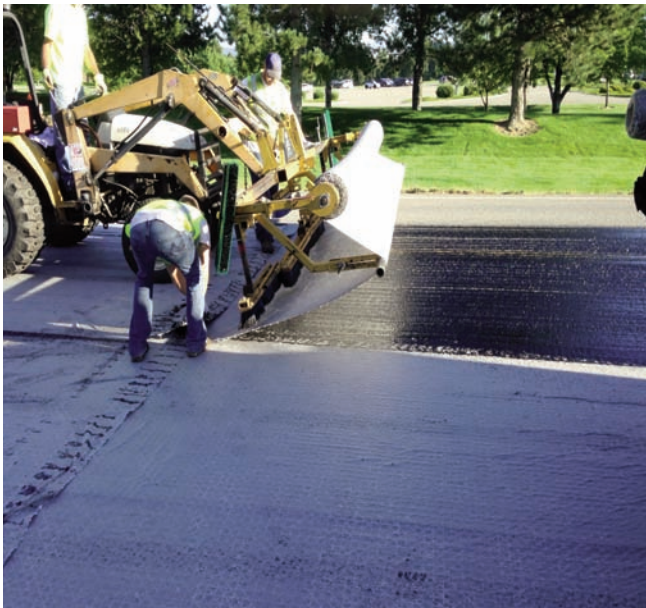
Above pictures: Installation of Mirafi® PGM-G 4 composite paving grid.
