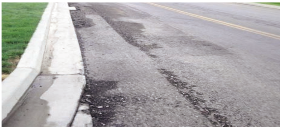
Above pictures: Mission Road before construction.
