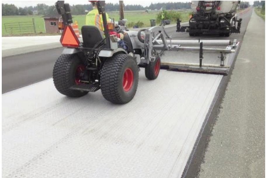
Installation of Mirafi® PGM-G 4 composite paving grid.
