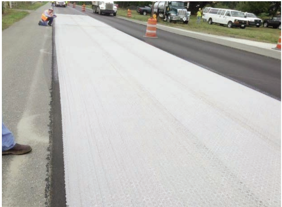
Installation of Mirafi® PGM-G 4 composite paving grid.
