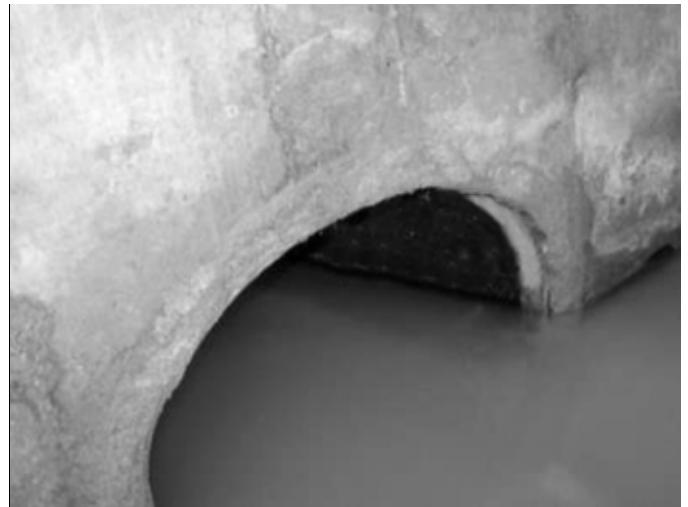
Example of a GOOD pipe installation. Pipe flush with the internal wall of the structure, clean grouting, and proper position.
