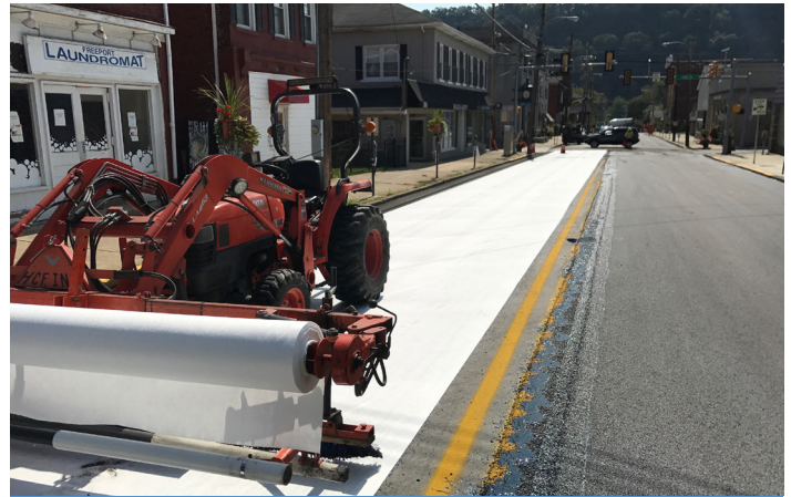
SOLUTION PETROMAT® Plus-White remains at a cooler temperature while creating a stress-absorbing interlayer
