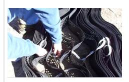
Figure 17 Threading Tendon and Attaching ATRA Tendon Clips
