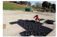
GEOPAVE units are installed in a herringbone pattern for multi-directional traffic.
