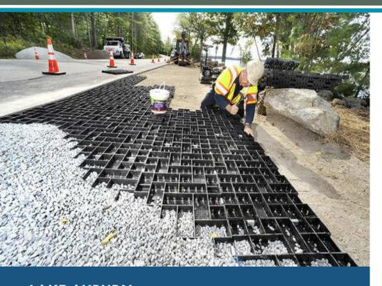
Highly-permeable GEOPAVE porous pavers meet storm-water drainage and traffic needs.
