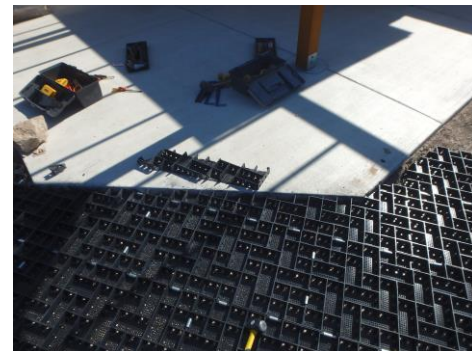
Figure 9 Joining GeoPave Units
