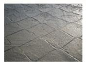
GEOWEB® slopes with concrete infill provide economical, hard-armored protection of slopes exposed to severe hydraulic or mechanical stresses. The quality,
