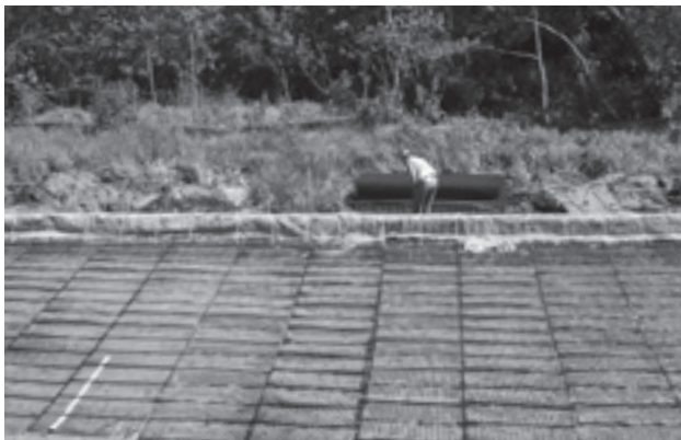
Installing the first layer of UX Geogrid perpendicular to the slope face.
