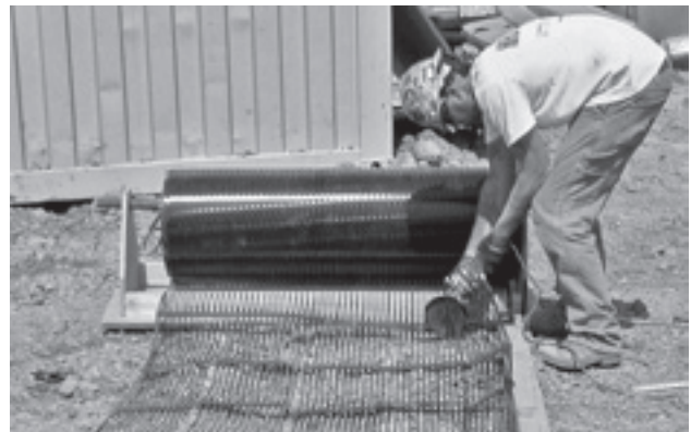
Field cutting the UX Geogrid.
