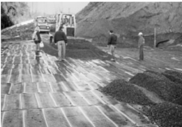
UX Geogrid and fill placement.
