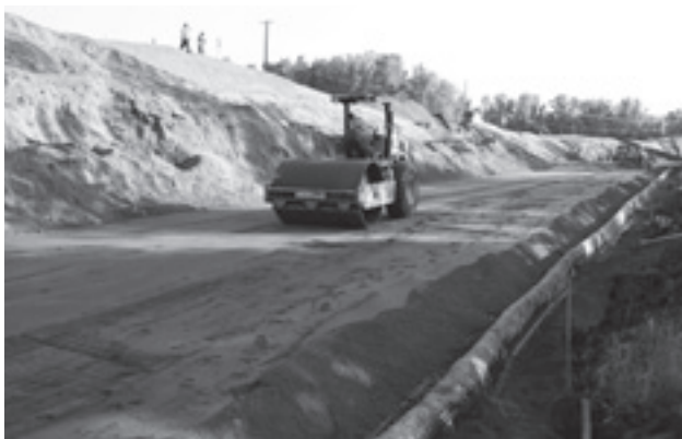
Heavy compaction equipment should be kept at least 3 ft from the face of the slope.
