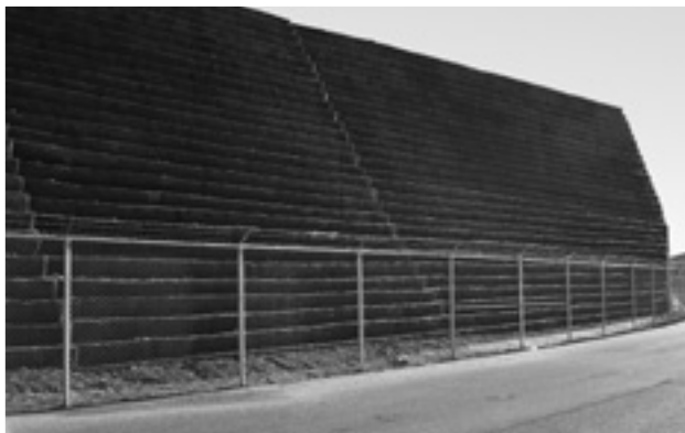
Sierra® Slope System installed, before and after vegetation.
