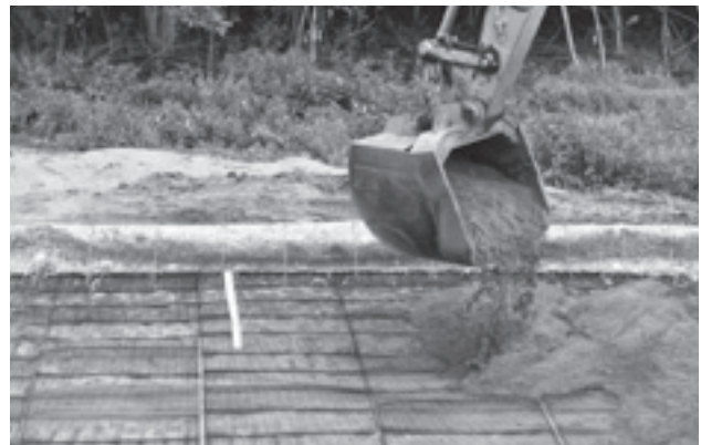
Fill should be placed and spread away from or parallel to the slope face.
